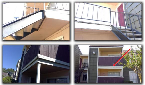
Damaged, rusted, and loose handrail/guardrails were found at many units. Damaged/cracked treads were also present. Repair is recommended.
