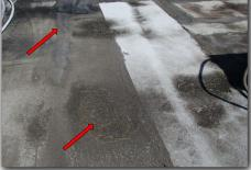
Worn asphalt was noted in areas of the flat roof coverings as evident by bare spots exposing underlying materials. Recommend further inspection/repairs by a qualified tradesman to prevent possible leaks.
