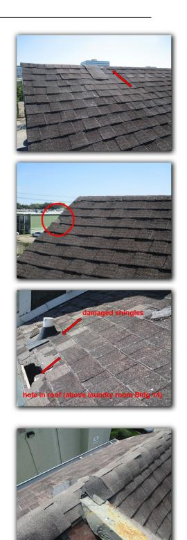
Exposed nail heads were found at roof jacks and / or sections of the flashings. All exposed nail heads should be sealed to prevent water penetrations.
