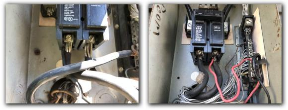
Oversized breakers were found within the electrical panel. Each breaker is rated for a specific size conductor. Ideally, these breakers should be re-sized by a licensed electrician. Including but not limited to the following locations:
