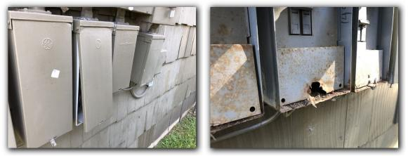
Many of the electrical panels are loose on the exterior wall of the building. The panels should be resecured by a licensed electrician. Debris (paint/texture, wood shavings, panel parts, etc.) was found within many of the electrical subpanels, main panels, and on various conductors. The interior of the panel and conductors in the panel should be cleaned as required by code.
