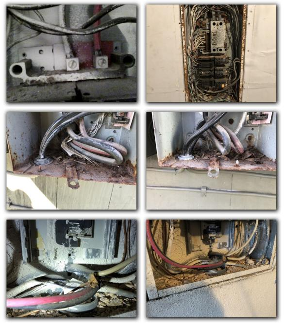
Corrosion was found at several conductors within the service panels indicating water/moisture penetrations. A licensed electrician should be consulted to correct these problems.
