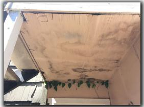
Evidence of improper support and/or damaged structural members were found at multiple balconies. Many of these areas appear to be structurally unsound. Evaluation of all stair/balconies by a Licensed Engineer and/or qualified tradesman for repair is recommended to prevent potential collapse and/or personal serious injury.
