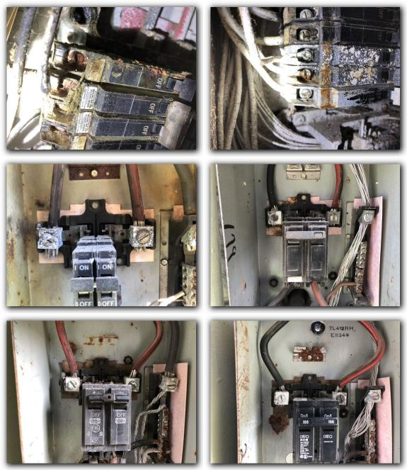
Many of the dead front covers are missing at the electrical panel. This is a safety issue due to the fact that all of the conductors are exposed when the cover is opened. A licensed electrician should repair this condition as soon as possible.
