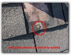
Deteriorated sealant / caulking was found at the rubber roof jacks. This material acts as a moisture barrier to prevent water from entering between boot and vent pipe. The re-sealing of the these areas should be considered.
