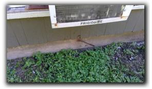
Exposed post tension tendon ends were noted at the visible portions of the foundation grade beams (B13). The steel tendon ends should be cleaned and covered with an approved material.
