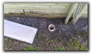
Standing water was found at the laundry room #2 exterior as evidence of improper plumbing drainage that may indicate underground breakage and or improper drainage. Repair by a licensed plumber is recommended.
