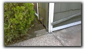
Missing conduit and improperly secured electrical conductors were noted in multiple units. Recommend evaluation for repair by a qualified tradesman
