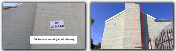
Diagonal cracking as evidence of potential differential movement
