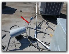
The conduit is loose at many locations of the exterior cooling unit(s) The conduit should be adjusted to completely cover/protect the conductors at this location.
