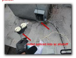
Exposed electrical connections were noted at various areas of the property. Improper electrical connections should be improved. All electrical connections should be made inside junction boxes fitted with cover plates.
