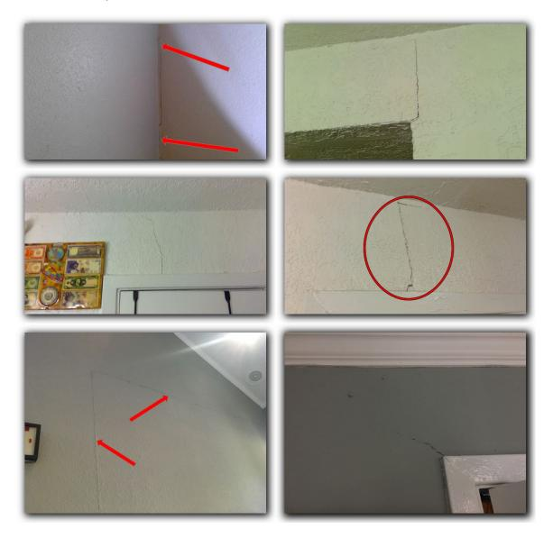
Damaged / missing areas were found at the interior of the units inspected The problems have been possibly caused by one or more of the following: water penetrations, insects, impact, foundation / structural movement, etc. Repairs should include replacement of damaged underlying materials where needed.
