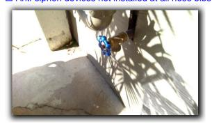
Items Damaged, Non-Functional, or Operating Improperly Exterior Missing hose bib / shutoff valve handles and leaking spouts were found at multiple areas.
