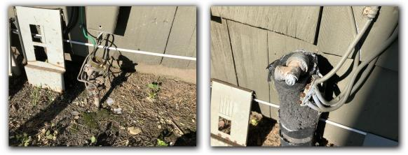
Many of the electrical meters are loose on the exterior wall of the buildings. The meter should be resecured by a licensed electrician.
