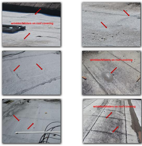
Alligatoring was noted on areas of the flat roof coverings. This can be caused by the suns UV rays that dry out any type of exposed asphaltic roofs. These areas should be monitored and repaired as needed to prevent future problems with the roof coverings.
