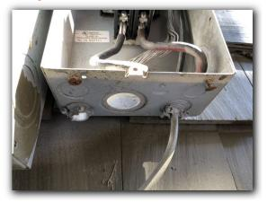
Many of the panel covers are bent, damaged, and loose. Recommend repairs or replacement by a licensed electrician.
