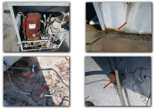
Missing and damaged panel covers were noted at most of the older systems. Recommend complete evaluation and repairs by a licensed HVAC technician.
