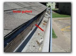
Leaky & damaged gutters were found around the perimeter of the roof coverings. The leaks should be repaired along with any damage caused by the leaks. It appears that multiple areas of damage have been caused by the leaking gutters. Repairs of the gutter / downspout systems as well as associated damages by qualified tradesmen is recommended.
