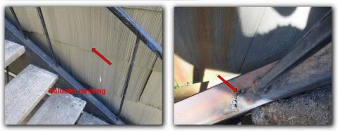
Rust, corrosion, damage and missing items were found at many of the handrails/balusters of exterior stairs. All rust should be removed to help prevent any future problems that may occur.
