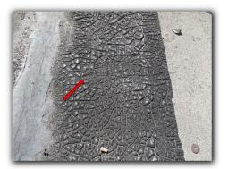
Soft spots were noted in a various locations on the rolled flat roofs. Soft spots on flat roofs could indicate rotted or improperly installed sheathing below the rolled roofing. A qualified tradesman should be contacted to inspect/repair the soft spots as needed.
