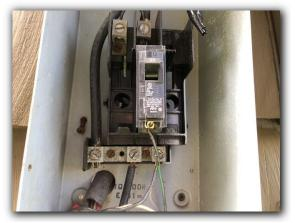
Most of the service box shows evidence of rusting, suggesting the presence of moisture. Many of the main electrical boxes are possible in need of replacement. Recommend further evaluation / replacement by a licensed electrician.
